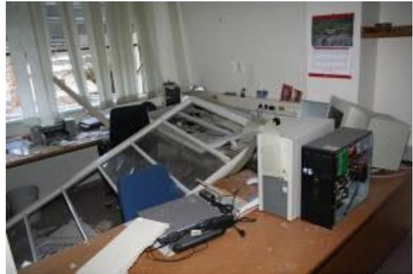
The upper photograph shows the effect on a normal window in the main office which was located at 240m from the explosion site. The main office suffered no serious structural damage, though considerable debris was scattered inside the building.
